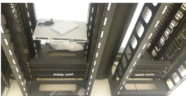
MONTAGEM RACK/RACK ASSEMBLY
