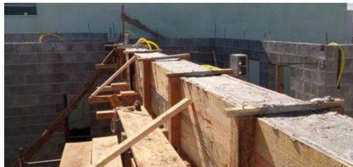
Figura 41 – Viga concretada – 30/04/2017
