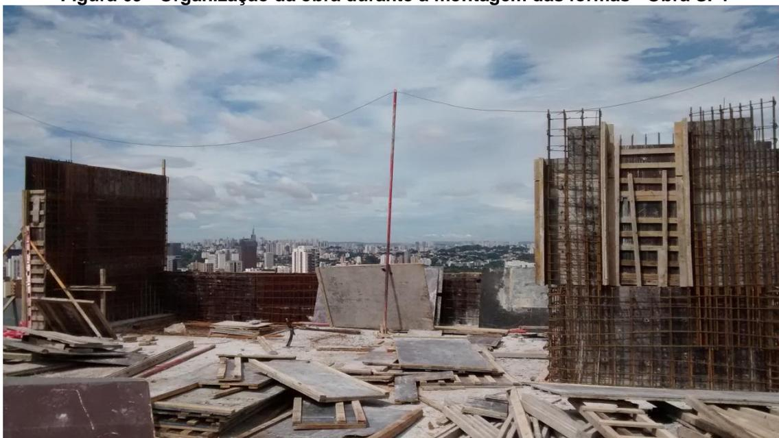
**Figura 70 - Fôrma da laje - Obra SP1**
